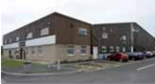
BUILDING CRAFTS TRAINING CENTRE St. Davids Close, Llansamlet, Swansea, SA6 8QT 01639 648120
